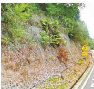
Rock face stabilised mesh
